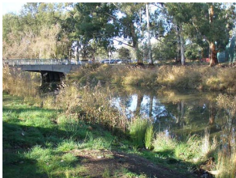
Figure 2. SUL765 on Sullivan's Creek, after weed removal, 2009.
