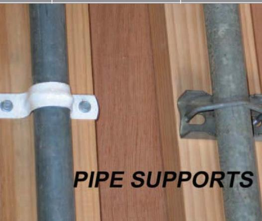
Figure 4: Fixing support pipes
