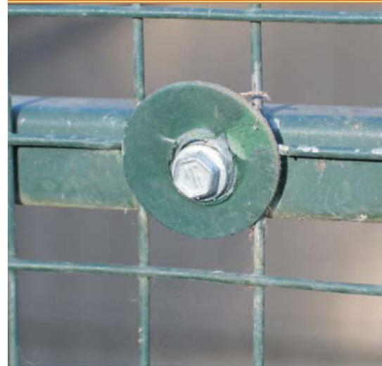
Figure 5: Fixing light mesh
