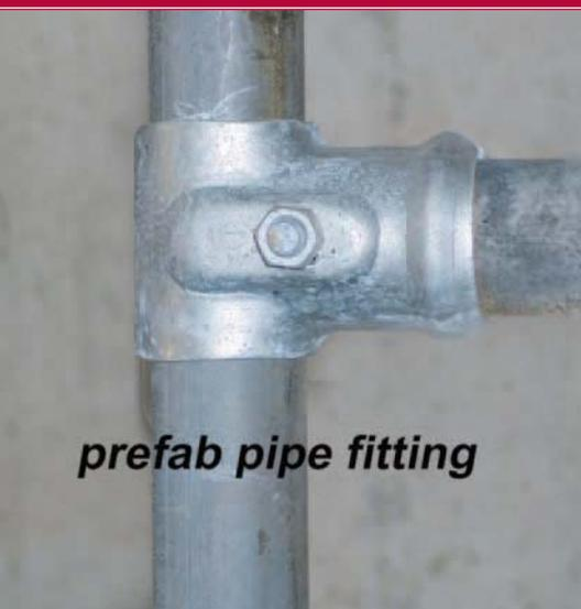
Figure 8: Prefab pipe fitting
